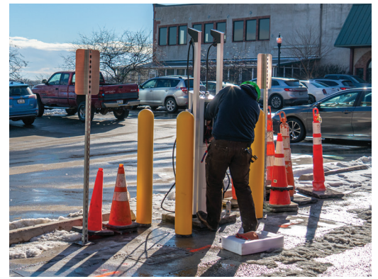
One of two new EV Chargers under construction
